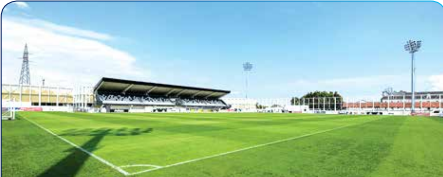
Figure 51. Example of floodlighting (International)
