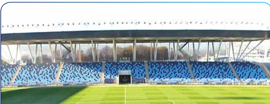
Figure 52. Example of a mini-stadium (International)
